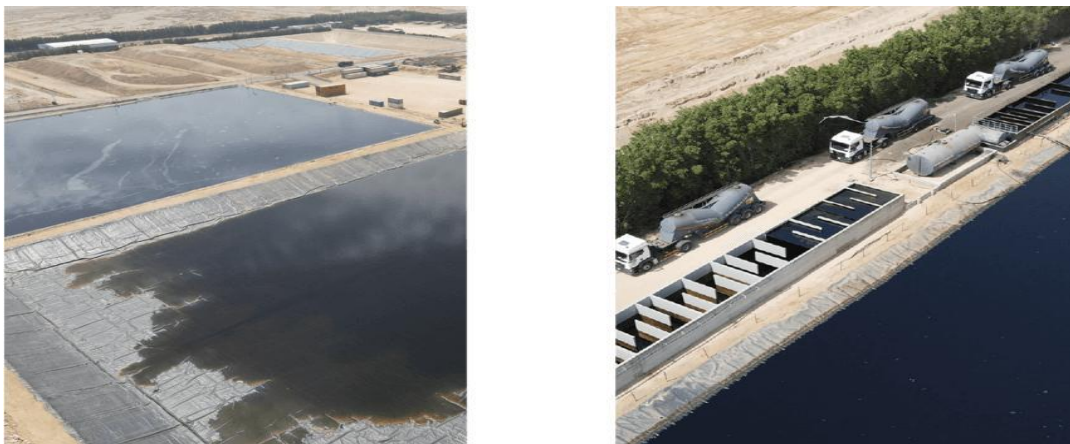
Figure 9. Kuwait's Lined Evaporation Ponds for Liquid Waste Management
