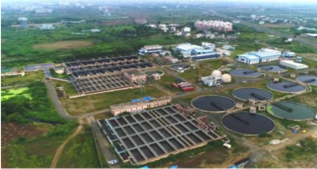
Figure 5 Represent Latest Advanced Robotic Technology for cleaning of Sewerage System Surat Municipal Corporation
